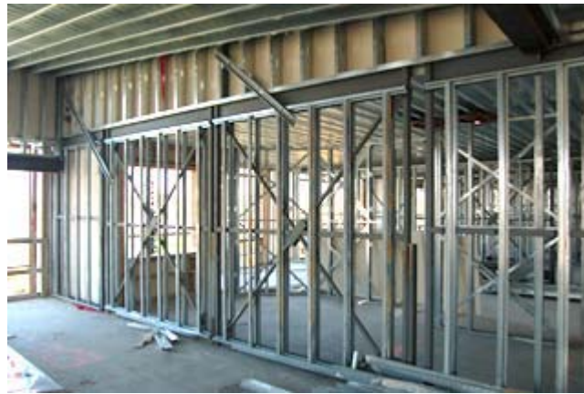
Inter Steel Structures Inc. used light-gauge steel to make the modular framing system, which can be covered up with finishes such as drywall.
